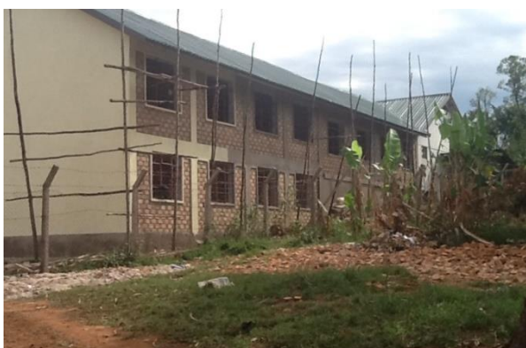
New library under construction at ESIIMI schools
